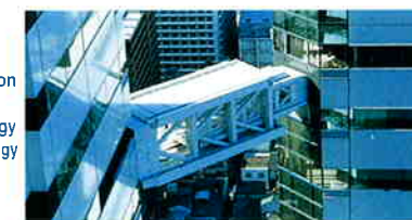
Active vibration control bridge applied to the three high-rise buildings located in Harumi Island Triton Square
