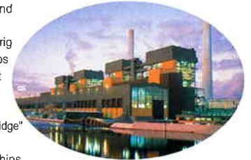
Boilers for Australia
